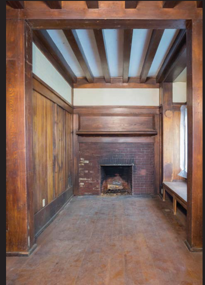
Interior Entry to be Restored- Phase 2
